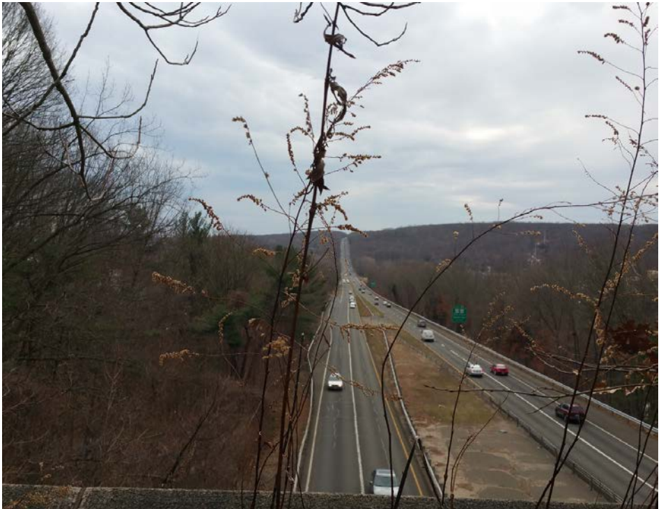
View from south portal looking south towards Exit 59
