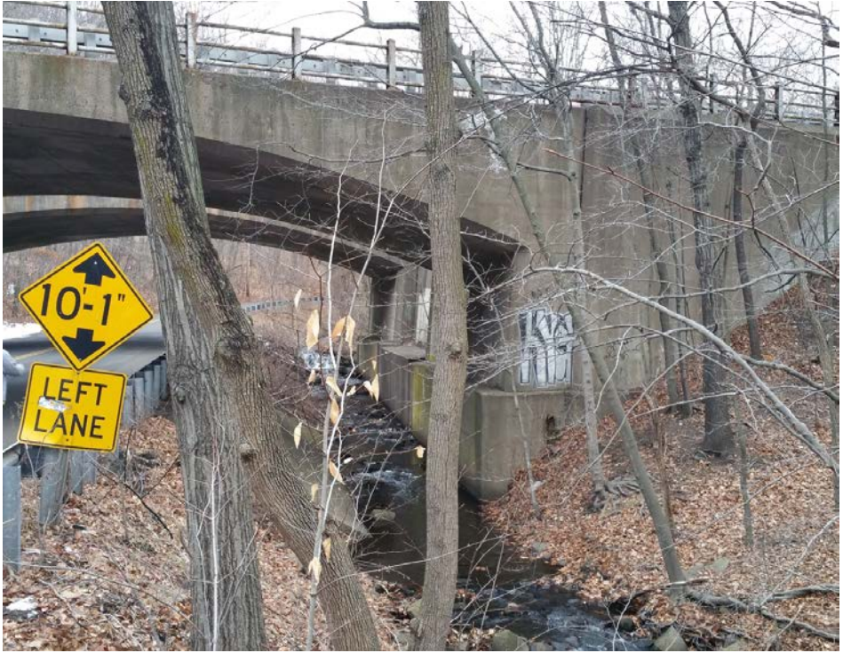
View of Route 15 bridges over Wintergreen Avenue and Wintergreen Brook
